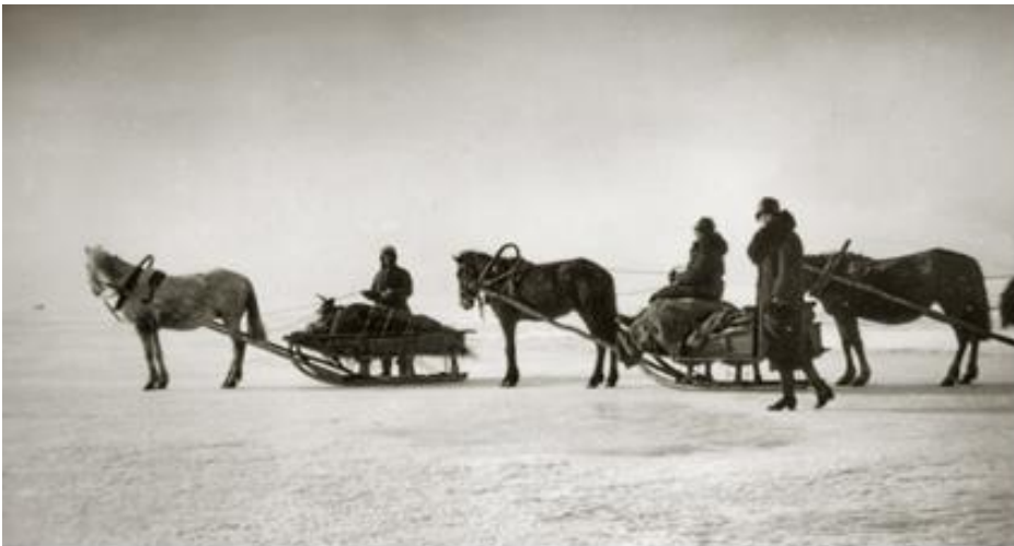
Figure 4. Ice road over the Baltic Sea from the island of Hiiumaa in 1930-ies. Photo credit Hiiumaa Muuseumid F9982.
